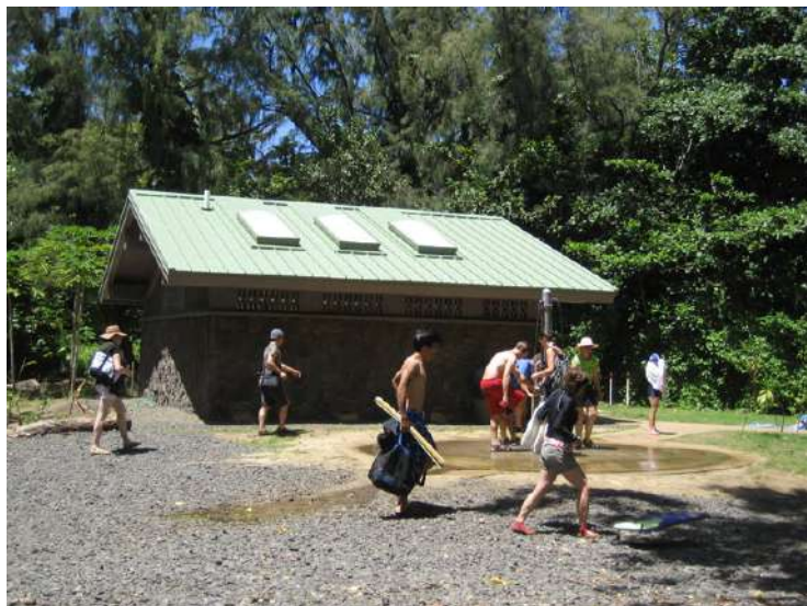
Photo 18 – New Comfort Station and Showers
